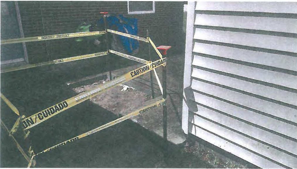
Picture 6: Site after completion of tank removal.
